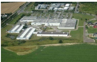
Capacity: 485KW Type: Rooftop Location: Magdeburg Germany
