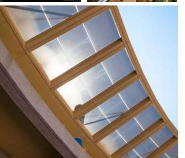
Polysolar's PS-M-NX opaque and transparent panels incorporate micromorph technology to achieve high efficiencies and aesthetic design.
