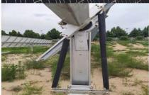
An independently developed tracking controller is installed to control the sun chasing rotation of photovoltaic parts by using astronomical algorithm + angle sensing to capture sunlight and maximize the power generation of the system
