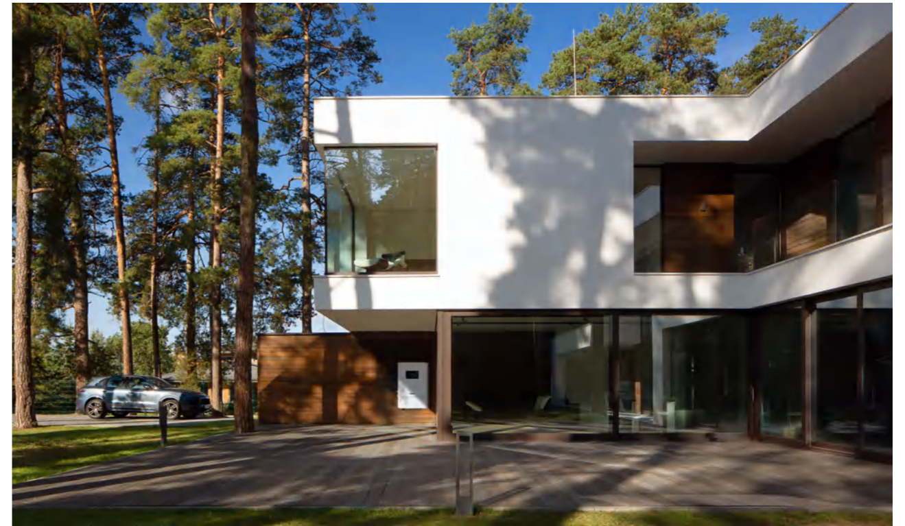
Residential Project in the United State 10kW
