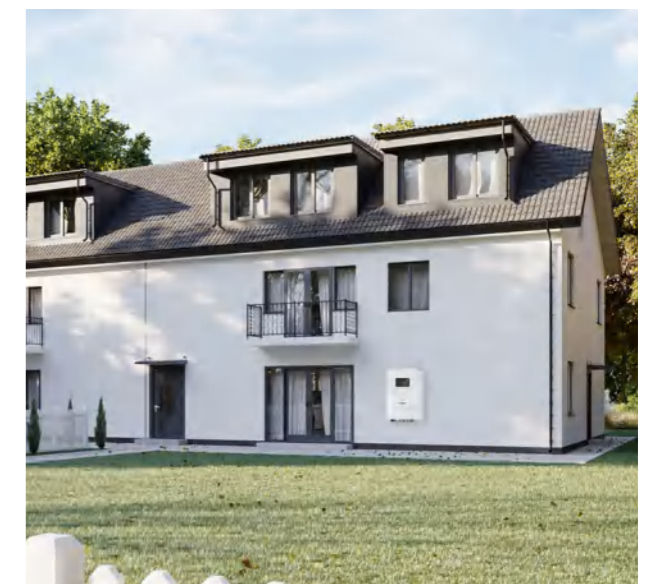
Residential Project in the United State 6kW
