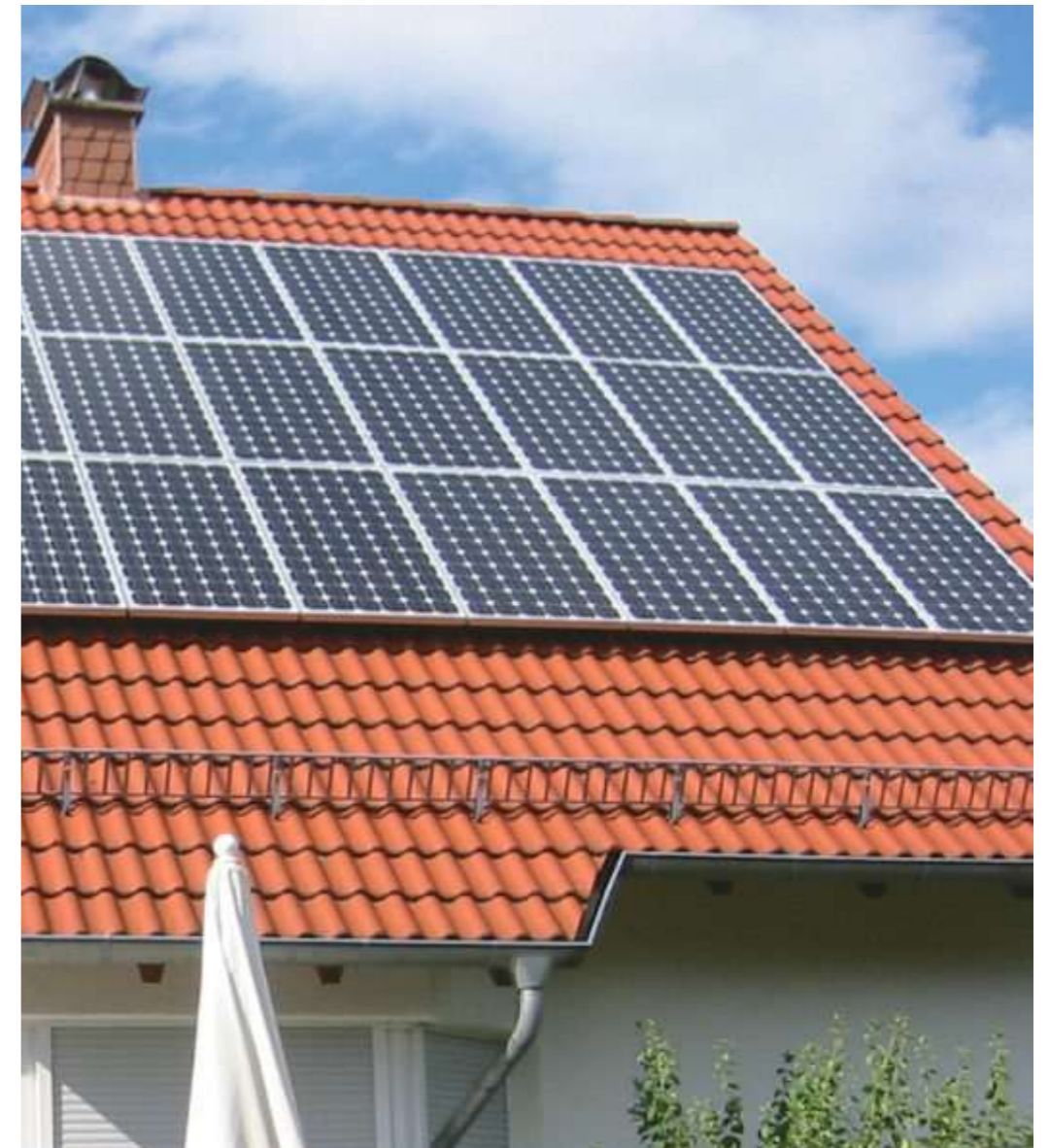
PV Rooftop Projects
