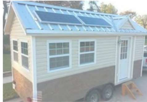
RV energy storage
