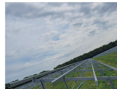
4 Install rails as drawing
