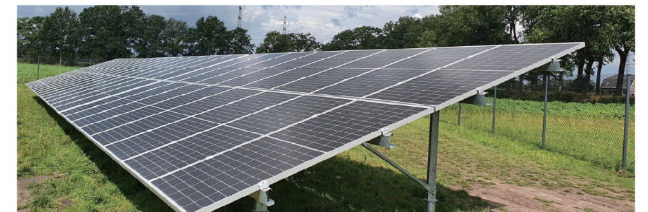
5 Fixing solar panel with mounting clamps
