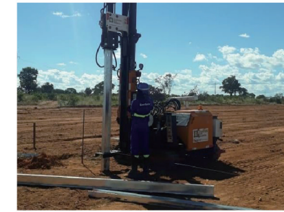
2 Ramming pile installation
