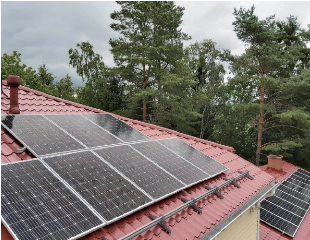
Finland, 6kW metal tile roof mounting
