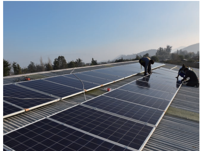
Chile, 16kW metal roof mounting
