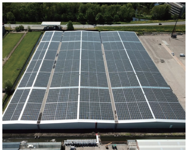
Guatemala, 2.8MW factory metal roof mounting
