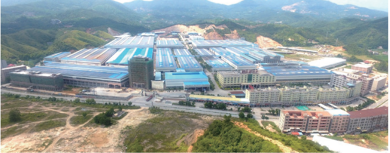
China, 11MW roof solar plant of our factory
