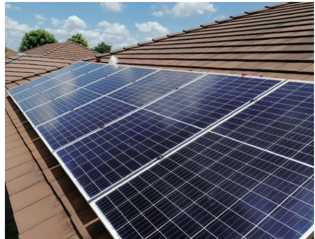
Thailand, 5kW tile roof mounting
