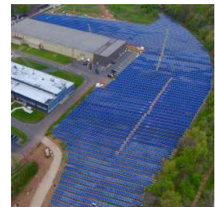
3.1MW - Bridgewater New Jersey
