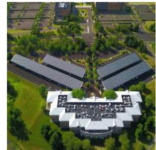
1.1 MW - HORSHAM PENNSYLVANIA
