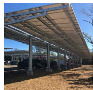
600 kW - VINELAND NEW JERSEY
