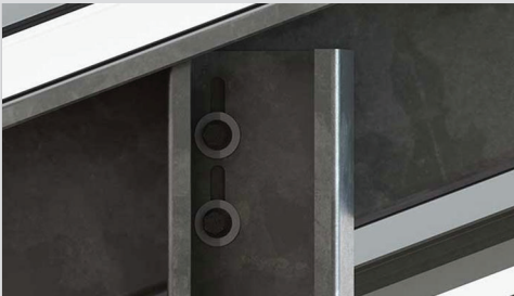
Slots enable vertical adjustability
