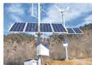
Base station/cell tower
