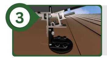
Assemble the second and additional rows of modules to the array with the patent-pending hook and loop feature with integrated bonding.
