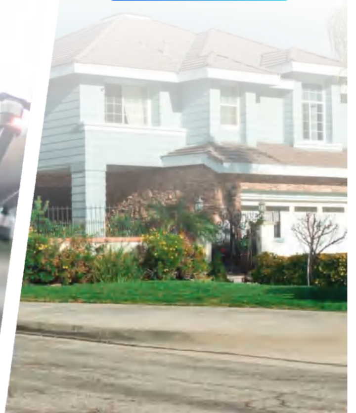
Home Backup Power
