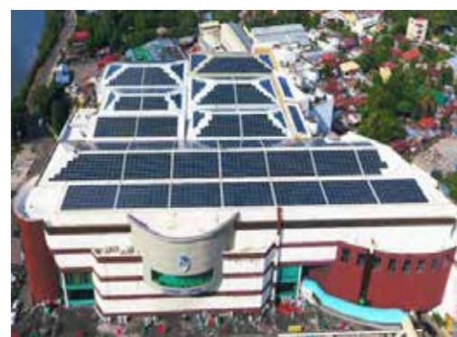
Project Location: Iloilo, Philippines Capacity: 1.9MWp Completion Year: 2016 Type: Metal roof Mounted
