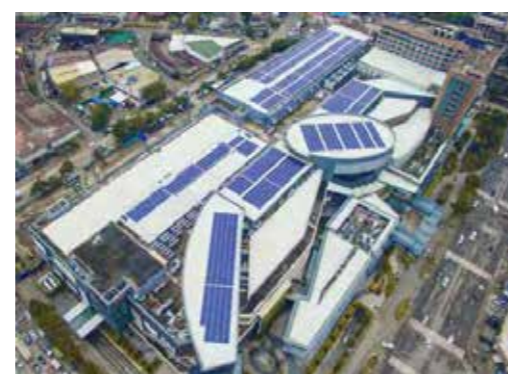
Project Location: Cebu, Philippines Capacity: 2.5MWp Completion Year: 2017 Type: Metal roof Mounted
