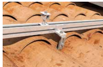
Pitched roof with tiles
