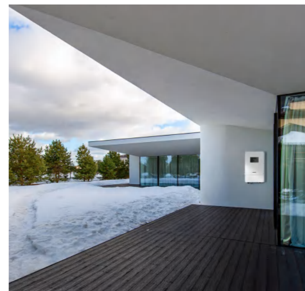
Residential Station Project in Utah 8kW
