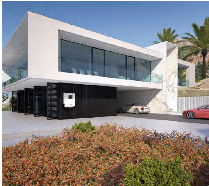
Residential Project in Sweden 12kW
