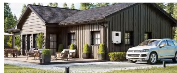
Residential Project in Germany 10kW
