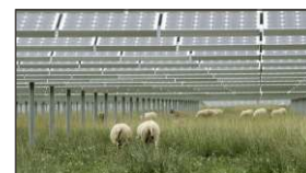
Farm solar generation system
