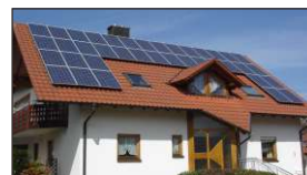
Off-grid home solar system
