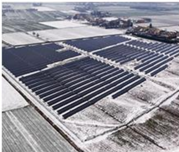
SALA BOLOGNESE (IT) ESPSA 185W, 2.5MW
