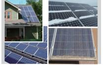
Nearby Shading, Soiling and inter-row shading
