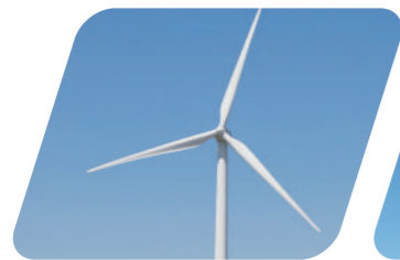
Wind Power System
