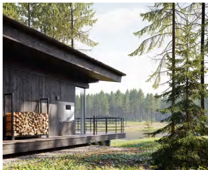
Residential Project in Estonia 8kW
