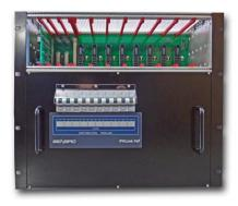
Under normal operation the ASR-25 regulators will be slave-switched by the ASR Controller in sequence to effect regulation of charge through the solar array stages into the battery bank(s).
