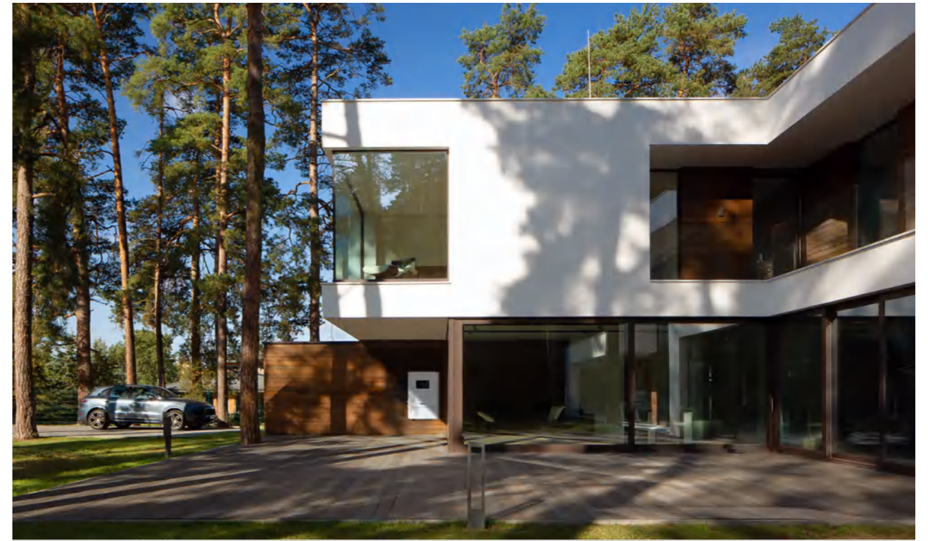
Residential Project in the United State 10kW
