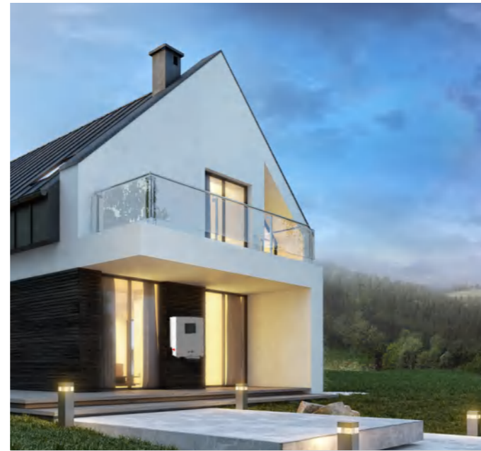
Residential Project in Germany 10kW
