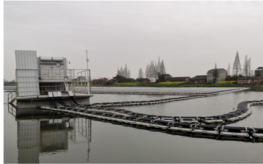
Equipment floater for cable from island to the shore
