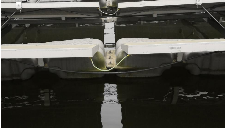
Module Grounding: using common ground wire
