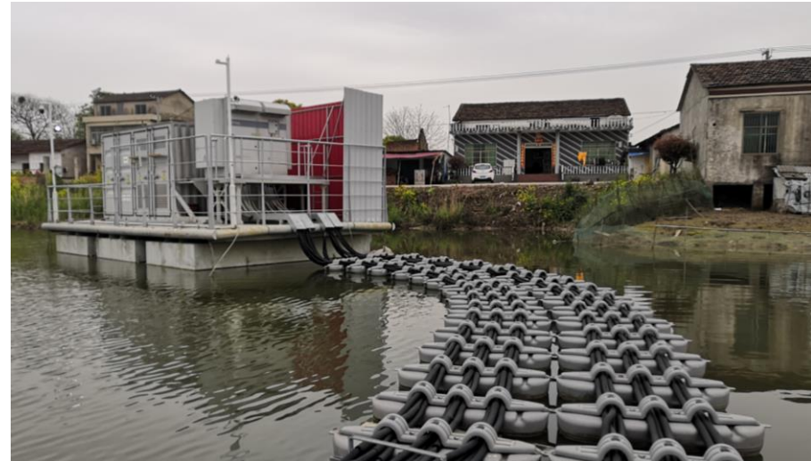
Cable floater for cable from island to the shore
