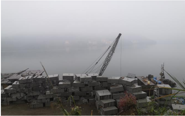
Step 1: Anchor Block Sinking
