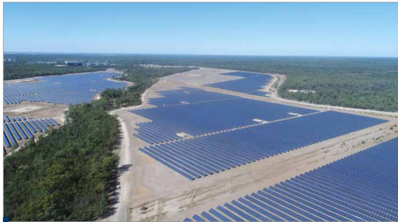
Darling Downs, Australia, 134 MW
