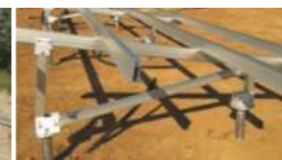
Ground screw foundation
