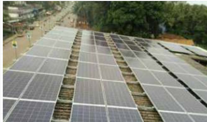
30kw asbestos rooftop at Udupi
