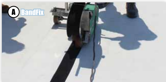
Installation of Bandfix on a synthetic membrane
