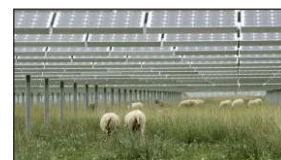
Farm solar generation system
